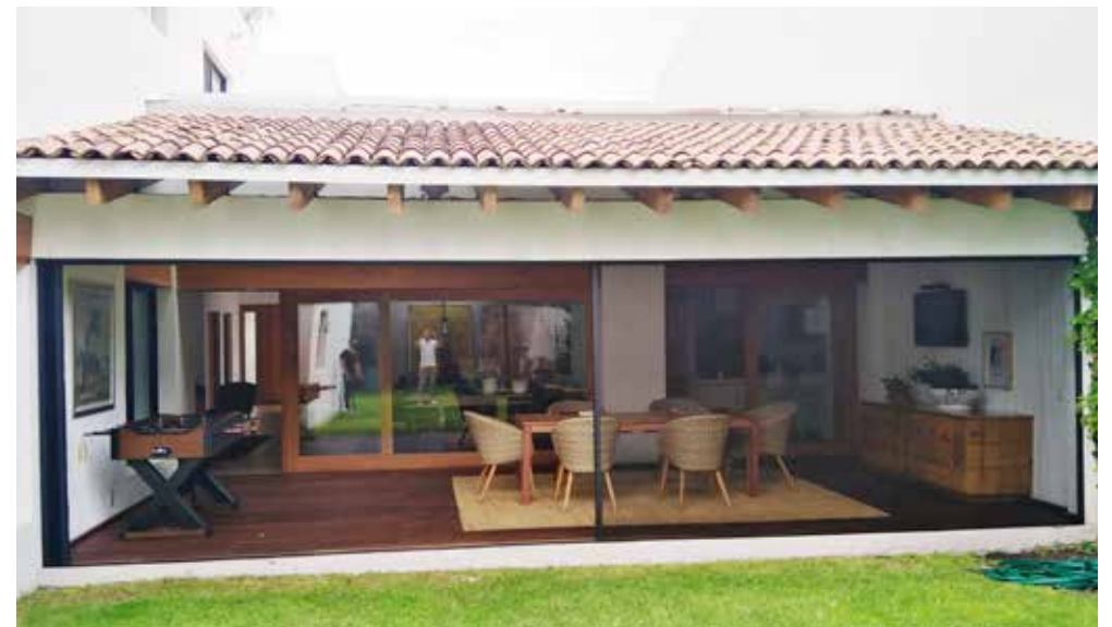
Half-open Fly-screen on the right side with central opening.
